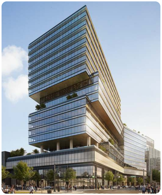
Reference image of Gateway Building
